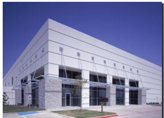
CORNER ARCHITECTURAL ENHANCEMENT
